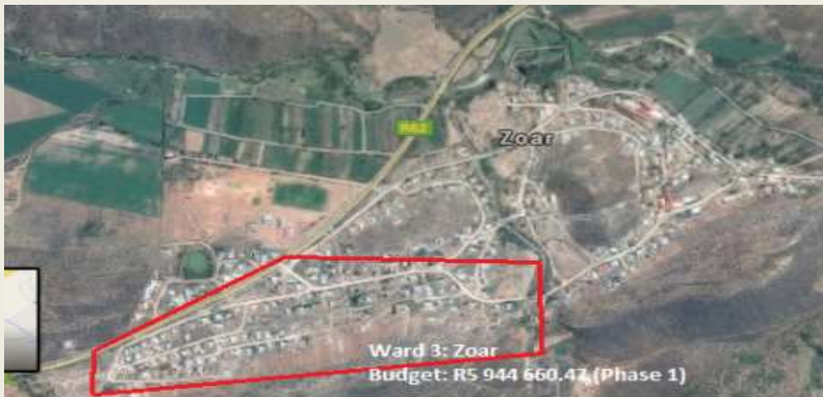
Figure 18: Zoar Internal Road upgrade
