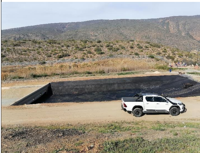
-Lining of Ponds
