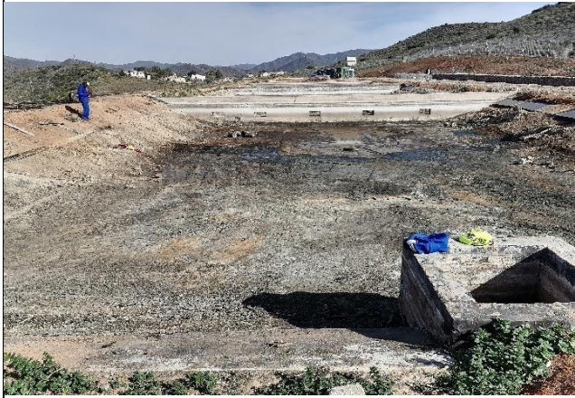
-Cleaning of Ponds
